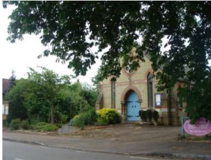
Picture 14 – Wesley Centenary Church, High Street, a fine example and representative of its type built in the late 19 th century: a potential candidate for formal listing.
