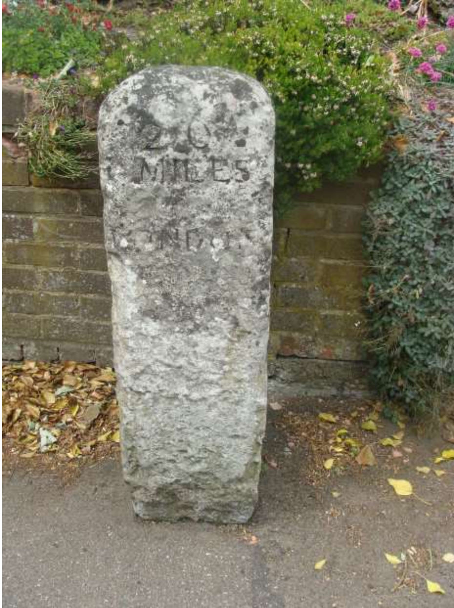
Picture 12 - Listed Milestone, cleaning, general restoration and repainting is recommended. It is included in the Council's Buildings at Risk Register.
