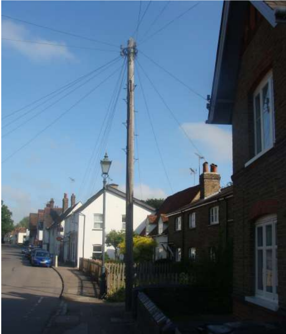
Picture 20 - One of several disruptive utility poles in the High Street.
