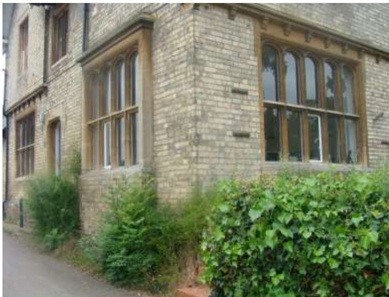
Picture 16 - Fine mullioned window detailing to nos. 92 - 96 High Street. Is there any local information as to the buildings original use?
