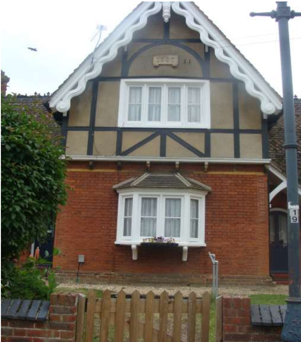
Picture 10 - 19 th century former Almshouses built by the Smith family. The decorative barge board detailing is found on other buildings elsewhere in the village.
